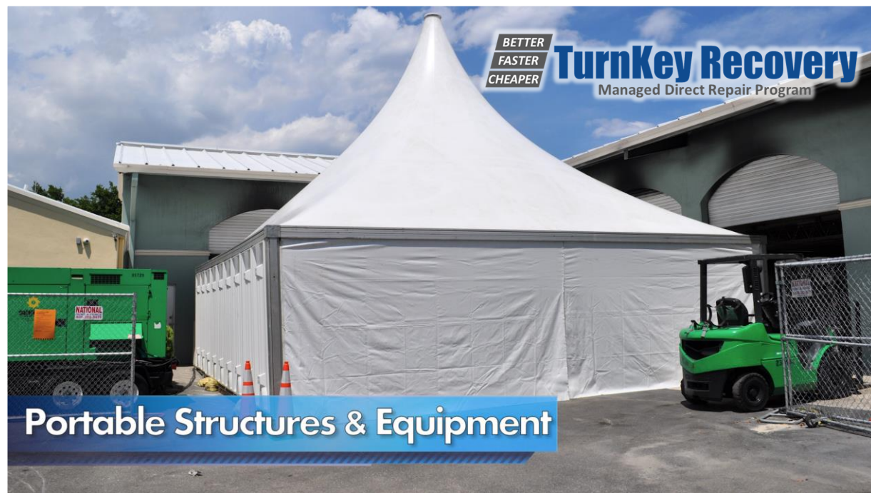
30x30 Low-Bay Structure, Fork Lift, 125KW Generator & 12ton AC Unit
