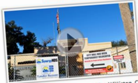
Williston City Hall Sinkhole Recovery
