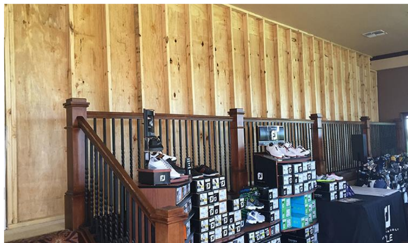
Power, HVAC & Board-Up
